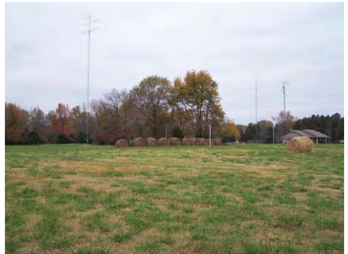
Figure 15 – 160 Meter Transmit Antenna (Left Tower)
