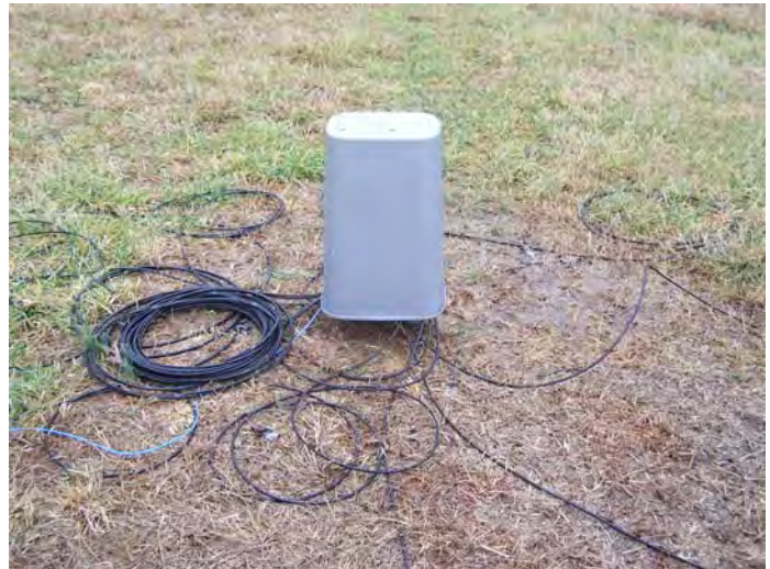
Figure 29: Completed Installation with Weather-proof cover
