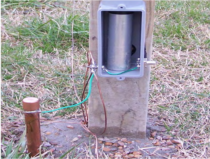
Figure 19: Ground Rod & Radial Attachment
