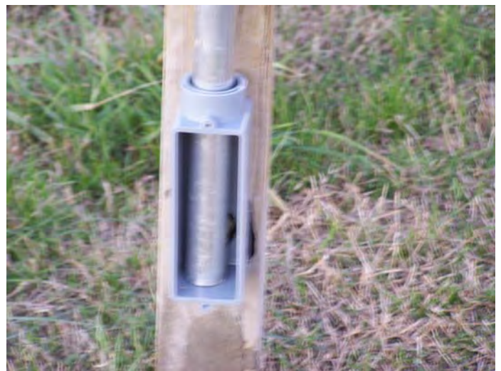
Figure 17: Vertical Element Sitting Inside Bottom Support Enclosure
