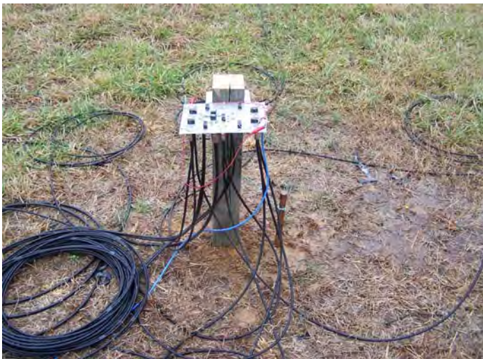
Figure 28 Installed Switching Unit at the Center of the Array
